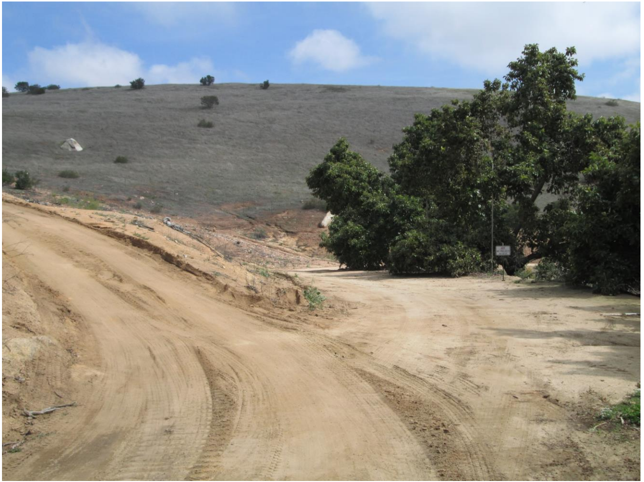
Photo 8: A “No Project Access” sign (photo, right) was installed at the junction of two existing access roads in order to ensure crews utilized approved exiting access roads.
